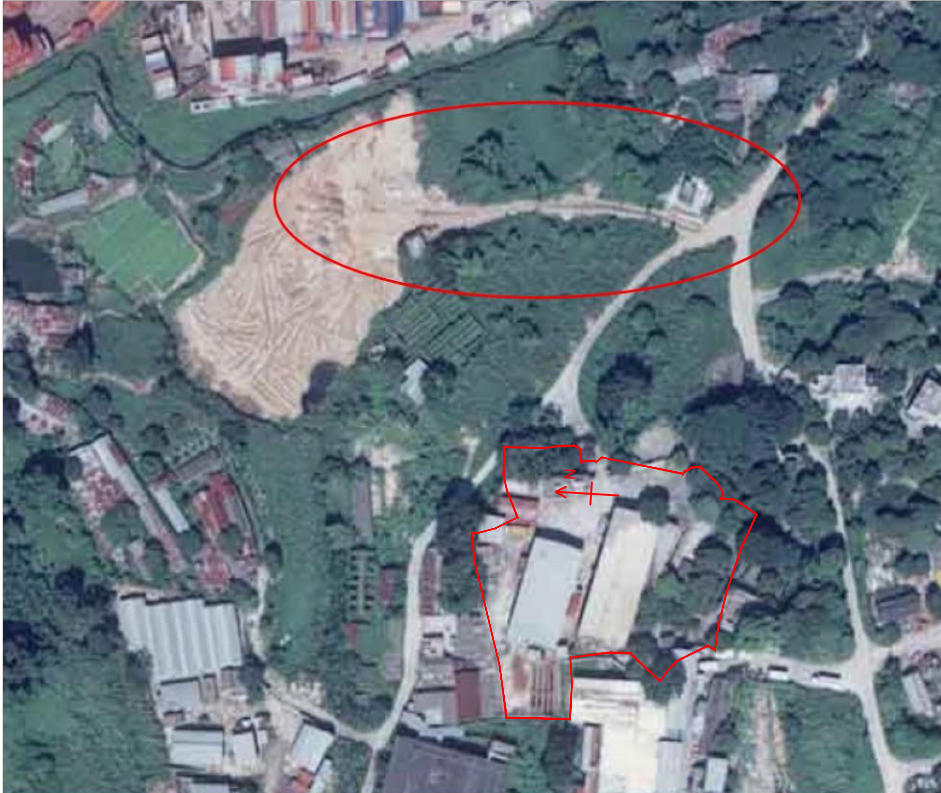
Plate 11 Year 1995 Aerial Photo shows U-Channel being constructed
