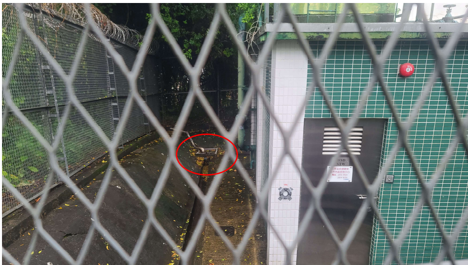
Plate 3 – Adjacent WSD Catchpit
