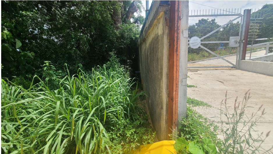
Plate 1 – The drainage runoff from the upper lot
