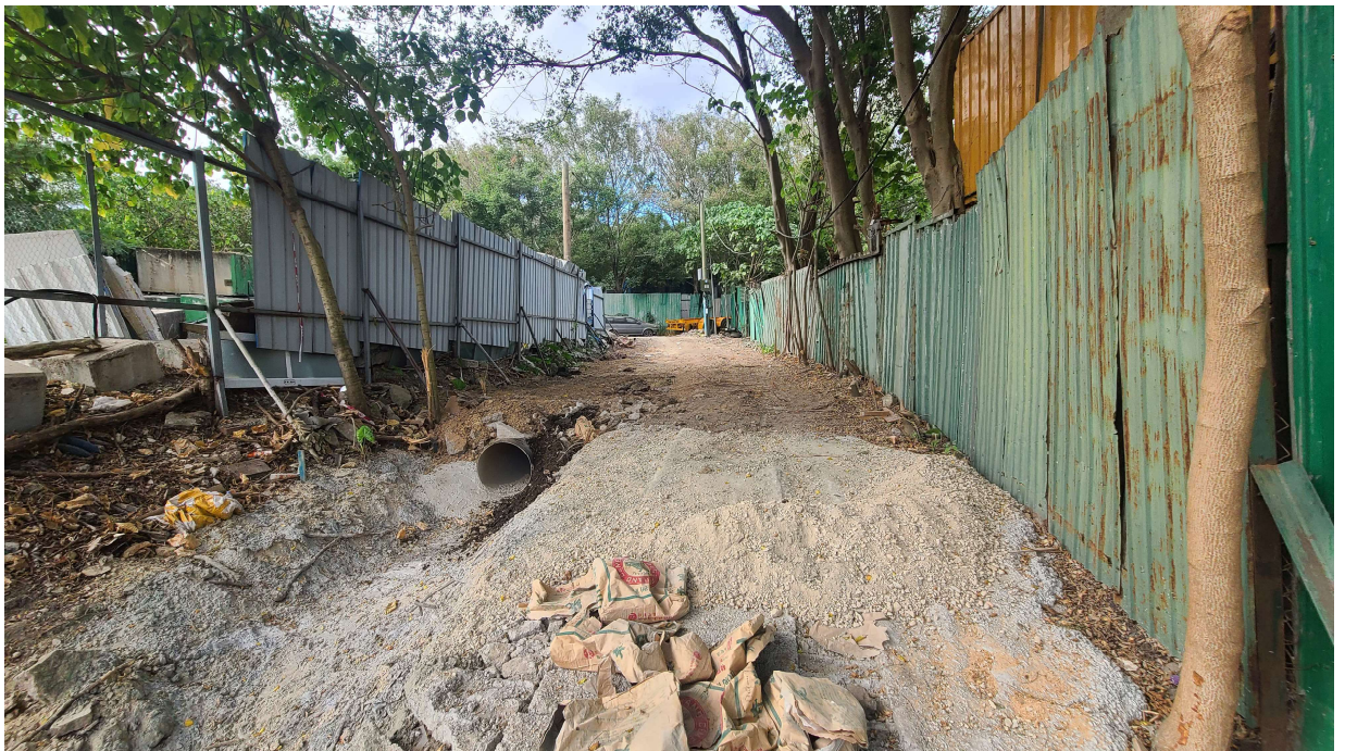
Plate 4b Existing Outlet in CEDD Site
