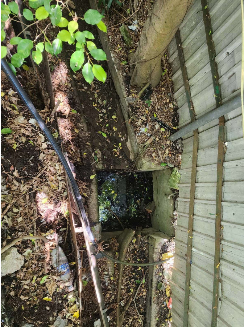
Plate 8 – Start of 600mm Pipe in Lot 50 (after cleaning)
